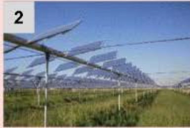
2 Castelvetro, Italy (source: www.remtec.energy )
