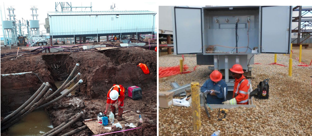
Figure 5: 25 kV three-phase underground feeders out of our Mowat Substation (left) and installing a pullbox and transformer at a customer site (right)
